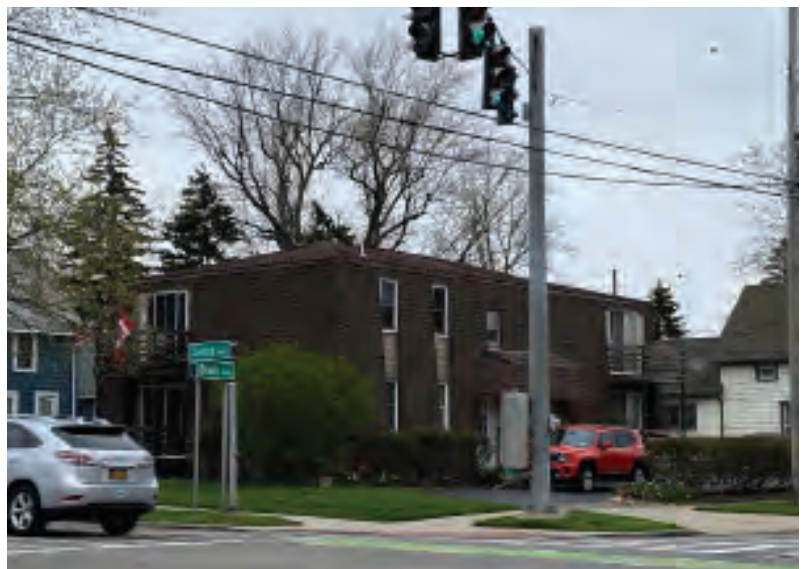
Fourplexes such as this building at Central Avenue and Brady Avenue can fit multiple units on a relatively small lot. (Mike Pesarchick, May 2022)
