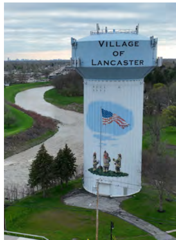
FIGURE 2-38: Water tower Source: Jordan Dawson, 2022
