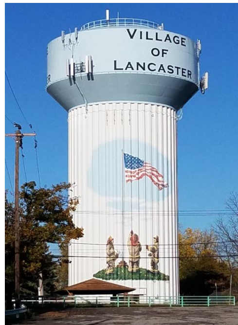
Village-Owned Former Water Storage Tank now Utilized to Hold Cellular Equipment
