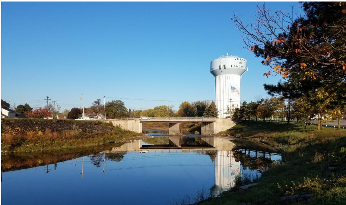
Cayuga Creek looking northwesterly towards the North Aurora Street Bridge
